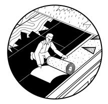
Position CCW EZRoof so that the end with the adhesive zip strip faces towards the overlap or top of roof.
